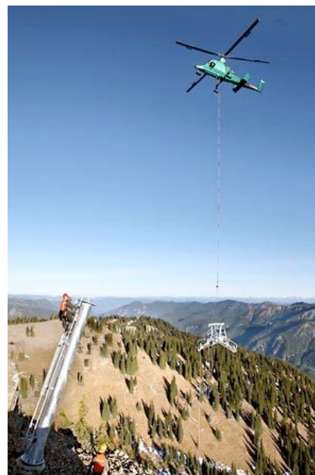
Kaman's KMAX aerial truck on a construction job.
